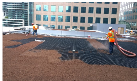
The extensive light version substrate is in accordance with the static requirements.
