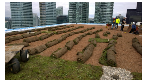
The high wind load requires additional measures to protect the System Build-up.
