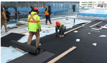
The Floradrain® FD 25-E elements retain rain-water to make it available to the vegetation later on.
